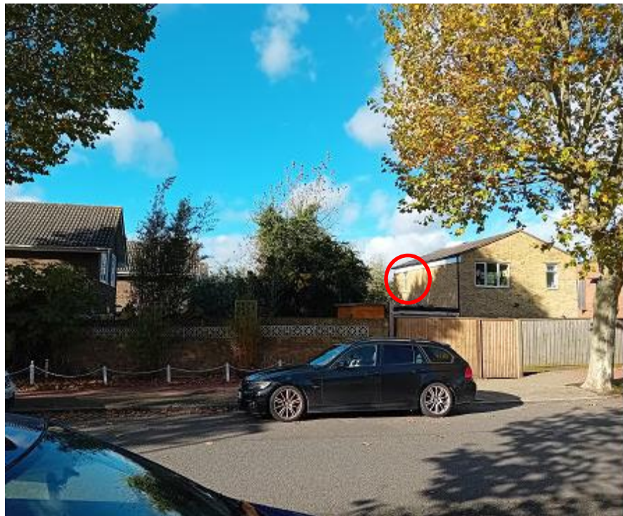
Figure 6 - First floor flank window facing Holmdene Close
