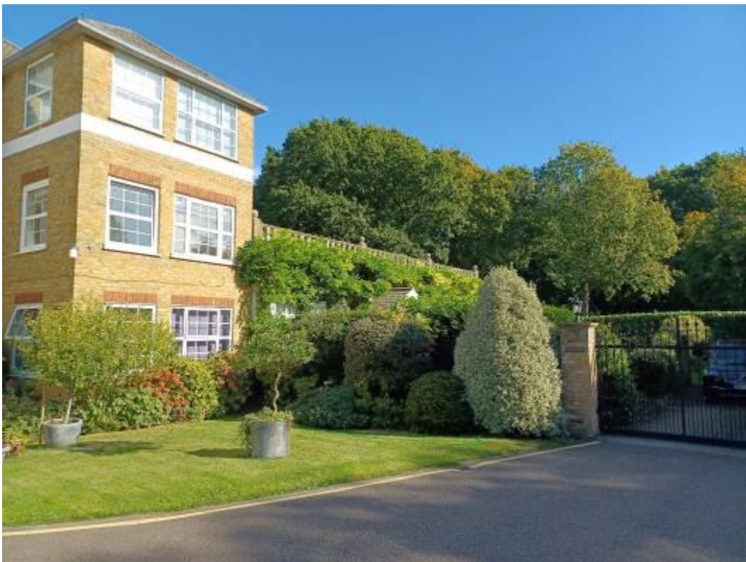
Figure 9. Flank elevation of Mulbarton Court and front elevation of Barton – showing parapet wall of flat roof but no solar panels visible
