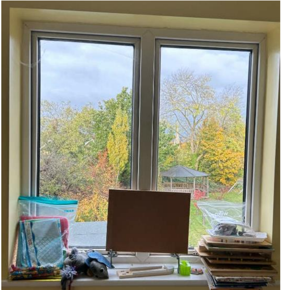
Figure 7 – Internal view from first floor rear window of pre-school
