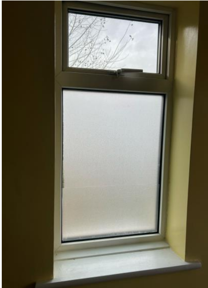
Figure 7 – Internal view from first floor flank window of pre-school
