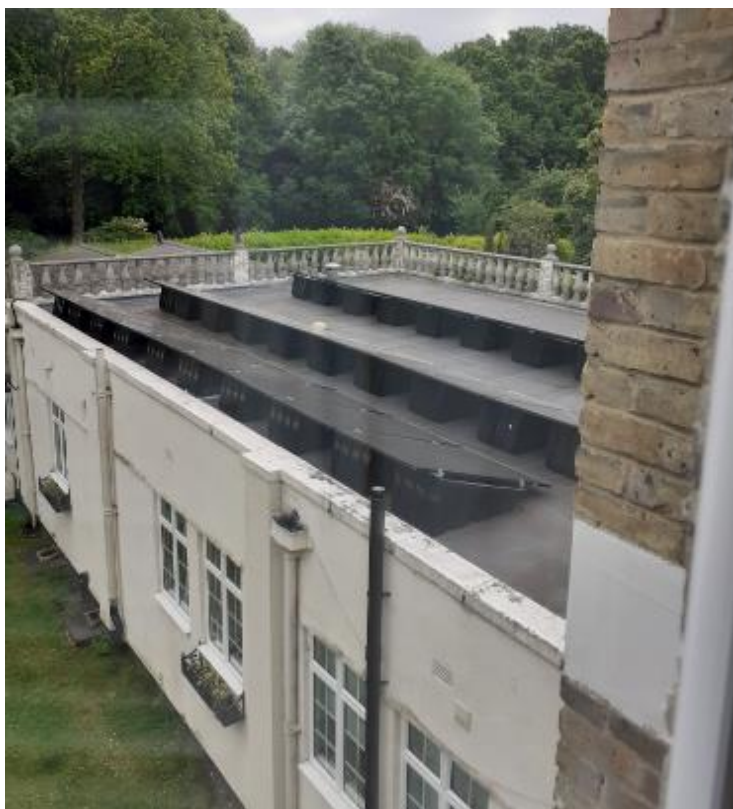
Figure 5. View of solar panels from window in Mulbarton Court
