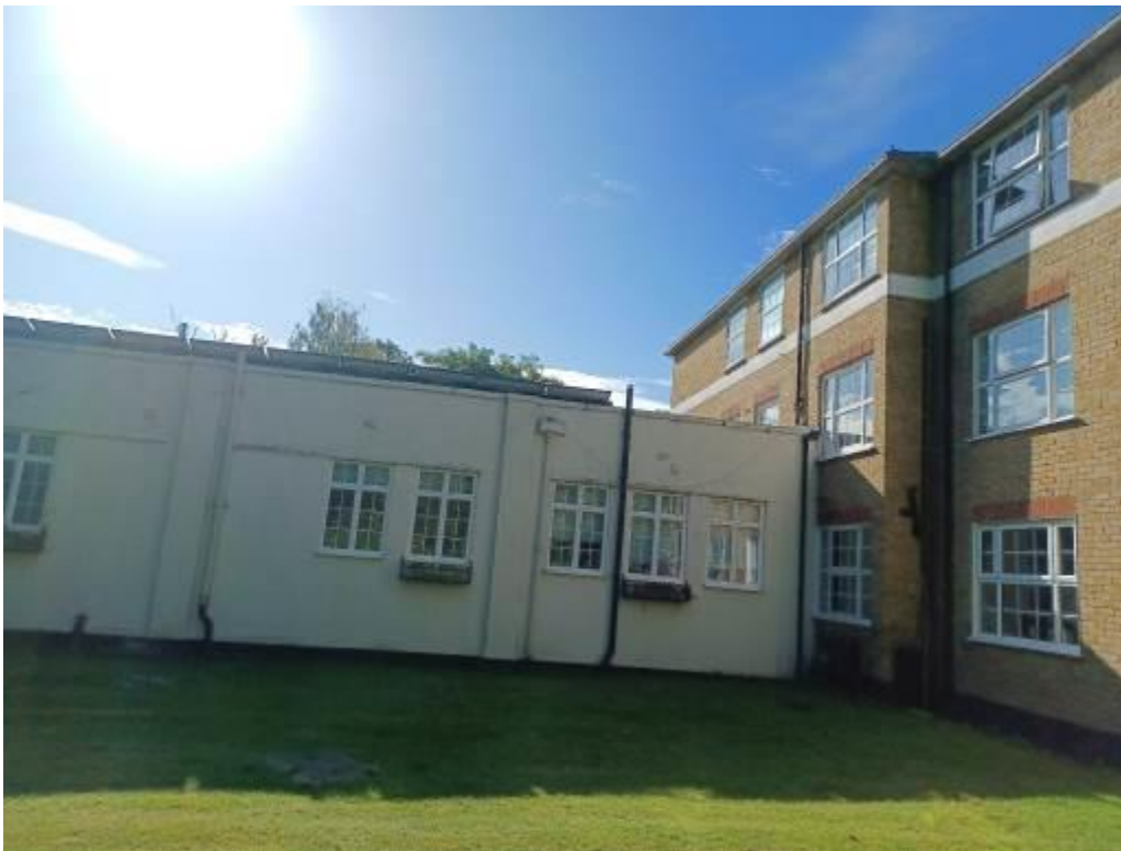
Figure 7. Solar panels viewed from garden and rear elevation of Mulbarton Court
