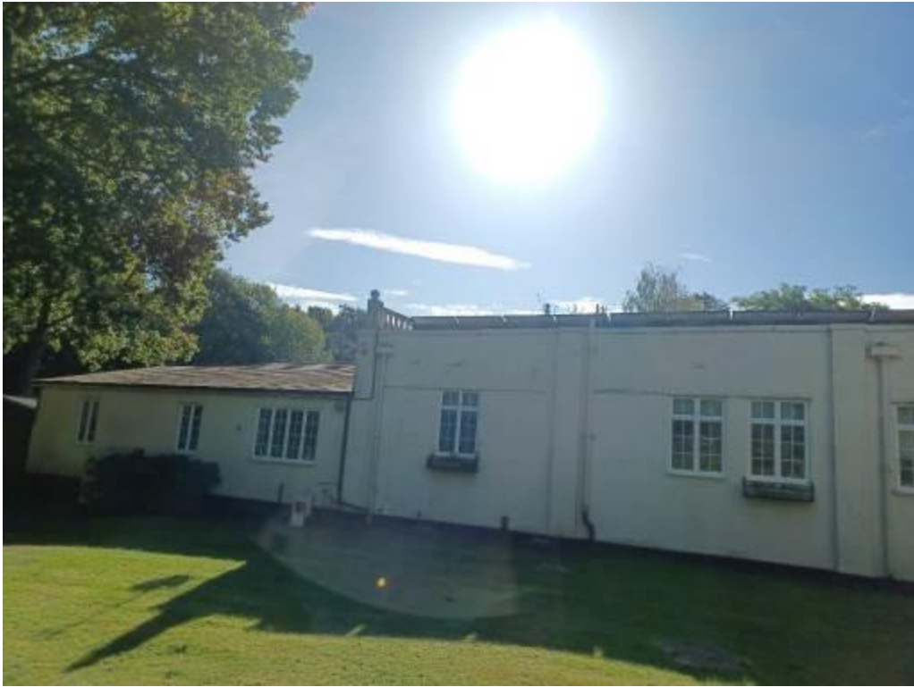
Figure 6. Solar panels viewed from garden
